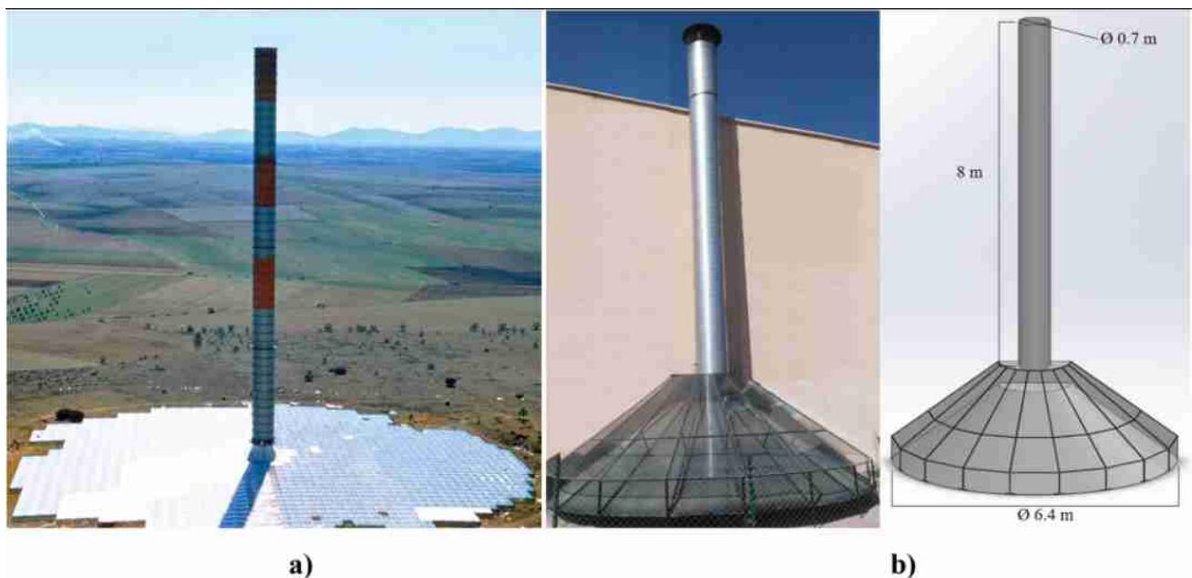
Fig. 2 a General view of the Manzanares prototype, b general and schematic view of the experimental setup
